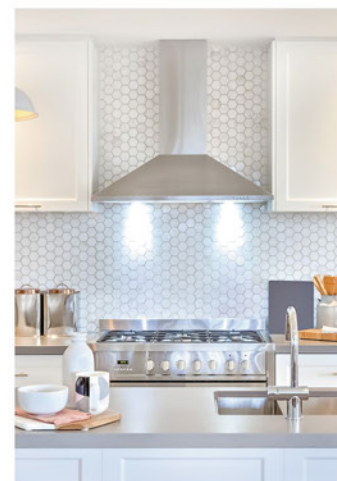
Kitchen Hood Exhaust
